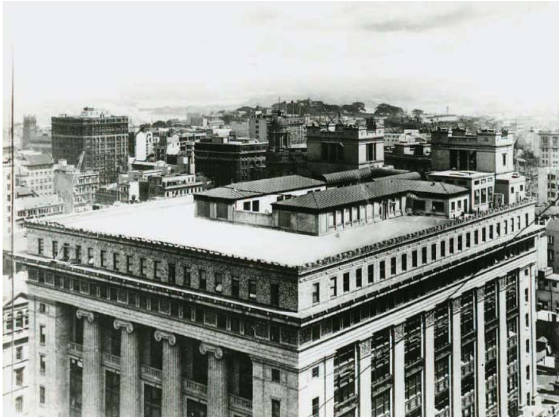
Figure 4 – Original configuration of structures on roof (c1928) – generally looking north-west
