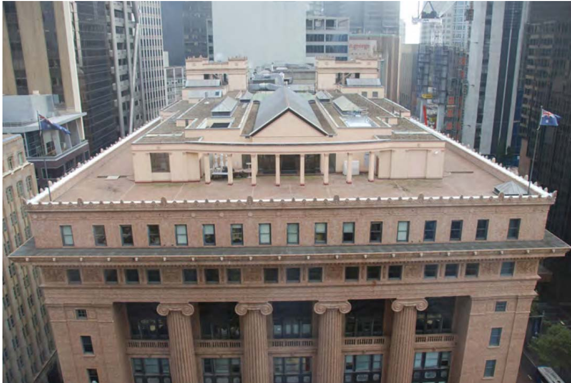
Figure 6 – View of 1980's rooftop additions (generally looking north)
